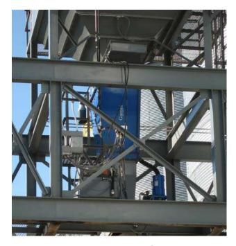
The Gamet 6800L Spout Style Sampling System is ideal for applications that require official sampling grades. It's a proven workhorse, with a reputation for reliability and performance dating back to the 1960s. Design is leak-proof and dust-free. A simple drive mechanism and the highest quality components ensure years of efficient, trouble-free operation.
